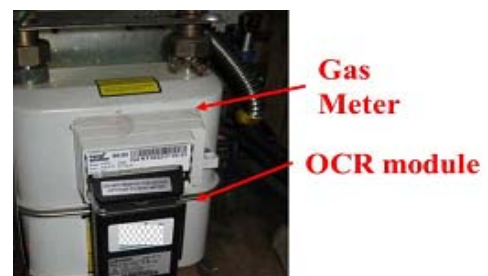
Fig.3: Traditional diaphragm meter with OCR module
